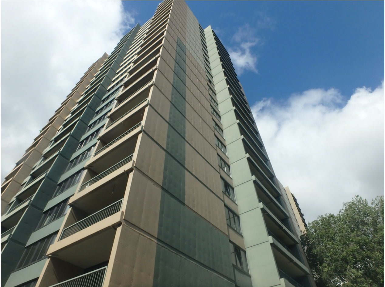
Overview: Rear Elevation
